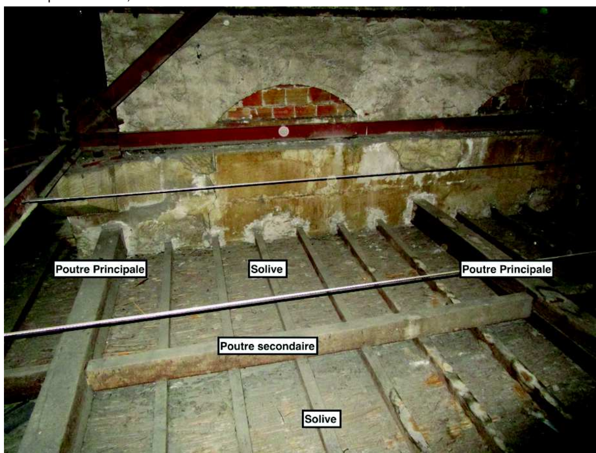
Figure 1: Ossature support du faux plafond
